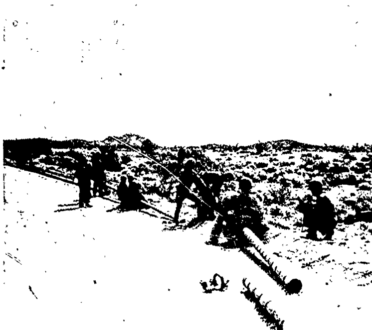
Four-man coupling crews at work putting in a portable pipe line. This pipe line went over a rise and down to water storage tanks of the Santa Fe Railroad, a distance of seven miles. (From the files of the Engineer Board, Yuma Test Branch)
