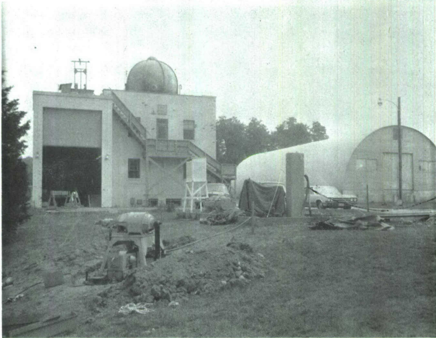
Fig. 1 - Test Site at the Chesapeake Bay Division. The photograph was taken looking south, and shows the vibration generator in the ground and Building 5 immediately behind it. The half-open overhead door in Building 5 leads into the Balloon Room, where recording instruments were installed and where some measurements of ground vibration were made. Photograph by Albert C. Grosvenor.
