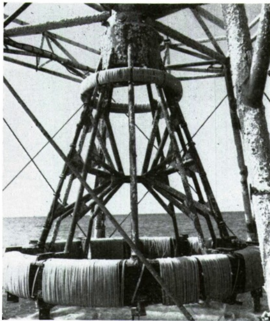
FIG. 4. The largest transducer element yet built, this 15-ton sound source was part of a facility at Eleuthera. Recovered under NUSC direction in July 1972, it was found to be still operable after six years on the ocean floor. Recording and analysis of data from the Bendix-built equipment were conducted at NUSC's Bermuda and New London laboratories.
