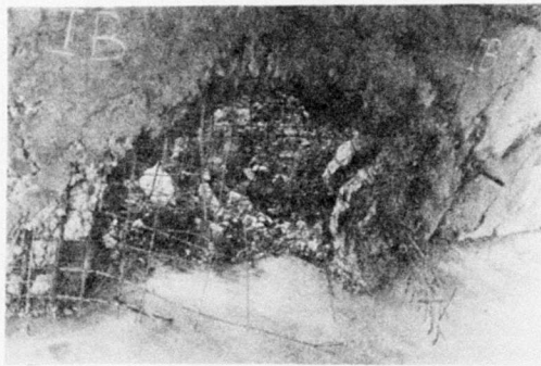
Fig 2b : Test No1 - inside damage
